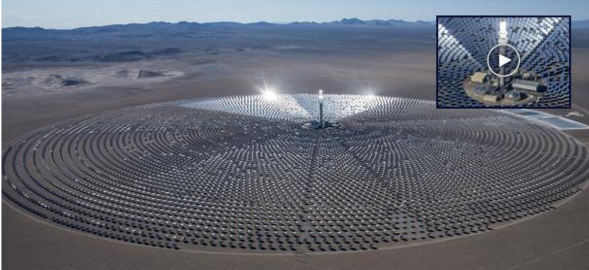
*SolarReserve's Crescent Dunes Solar Energy Facility, in commercial operation in Nevada USA, delivers both 110 megawatts of power plus 1,100 megawatt-hours of energy storage*
